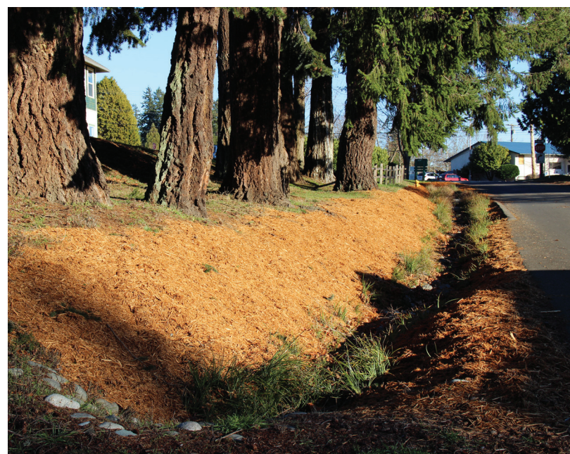
above: existing biofiltration swale and large trees
