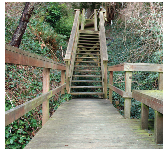
above: beach access stair
